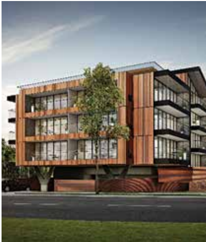
Built with eternity in mind, k20 Architecture's Eternity Life in West Footscray is the largest residential timber building in Victoria
