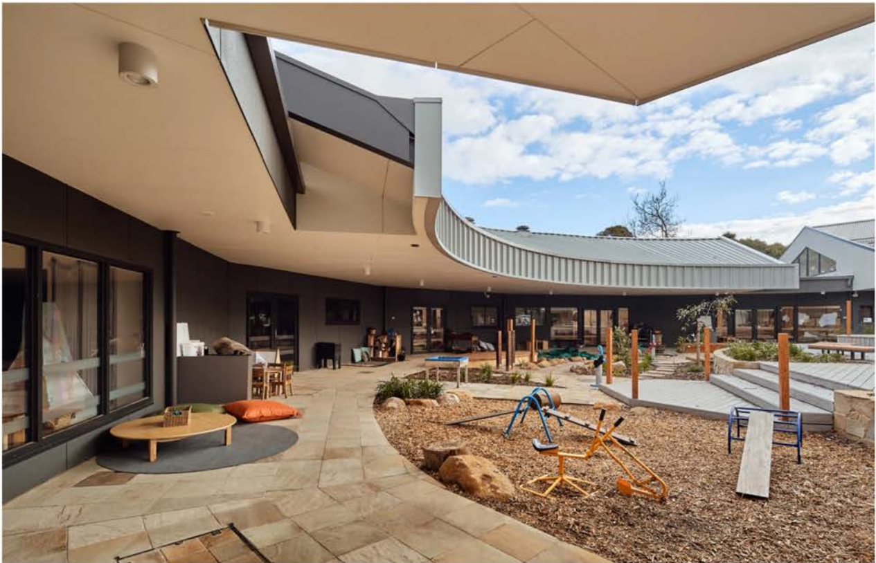
The Bayswater Early Years Hub's exterior has some shaded areas to relax while keeping an eye on the kids at play Peter Bennetts
